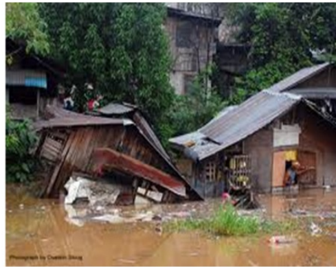
Storm effects on housing/settlement
